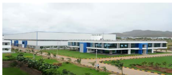
ACG-Lukaps facility, Ludbreg
